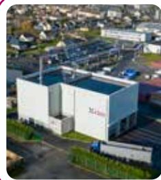
Commissioning of a carbon-free steam production for the Bel factory in Evron.
