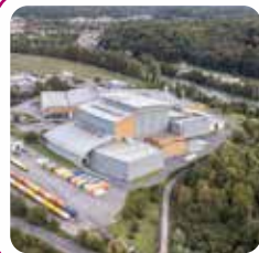
The inter-municipal syndicate of the Oise department entrusts Idex with the construction of a third line at the Villers-Saint-Paul energy-from-waste unit.
